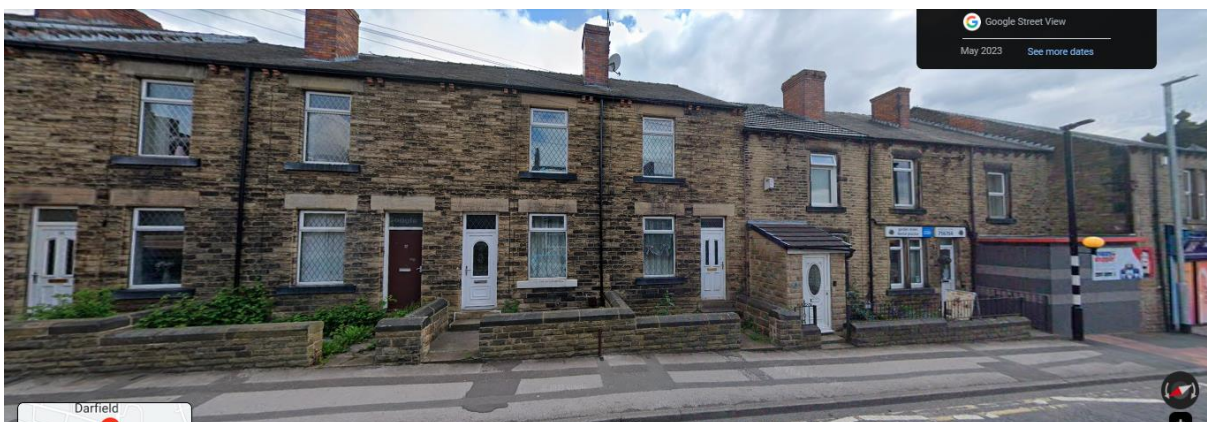
Figure 2. Opposite side of the road to Kosta's Place, showing minimum five residential properties in the immediate vicinity.
